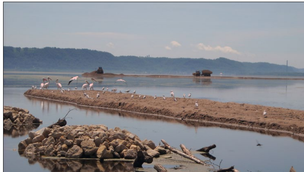
A rock log structure connecting two islands at the Pool 8 Islands project near Brownsville, Wisconsin, June 22, 2010. USACE courtesy photo
